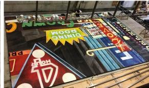
For As You Like It at Royal MTC, the scenic artists were given a digital collage with measurements. They used a grid system to scale it up, drawing it all onto a huge, stage-filling backdrop. To get an idea of the size, look for the tiny scenic painter in the third image! (Set design by Pam Johnson)
